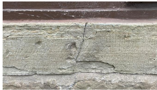
Left ground floor window to westerly elevation - cracked left side jamb and cracked cill.
