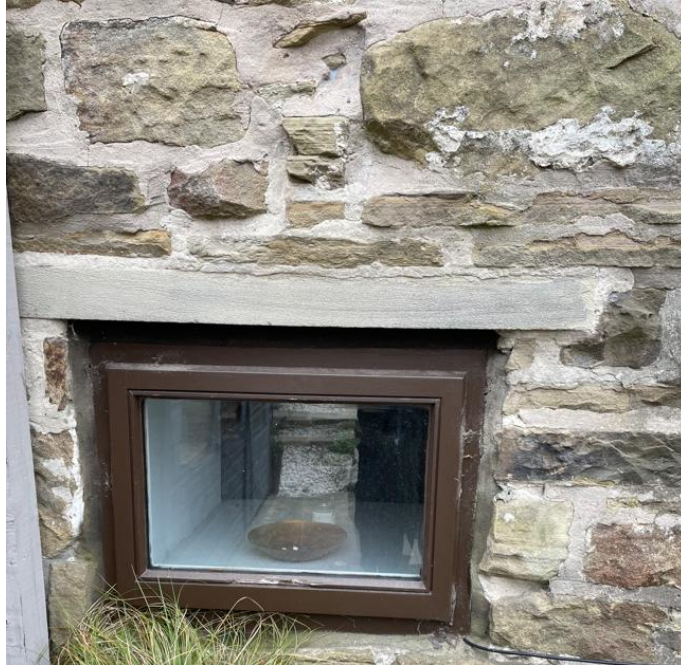
As it currently is with hard cement mortar
