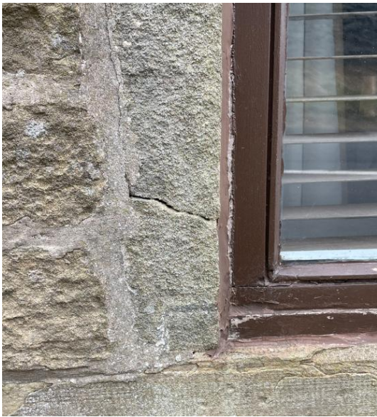
Left ground floor window to westerly elevation - cracked left side jamb and cracked cill.
