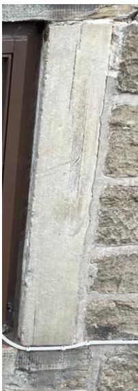
Right, ground floor window to westerly elevation - splitting to right side jamb and cracked cill.
