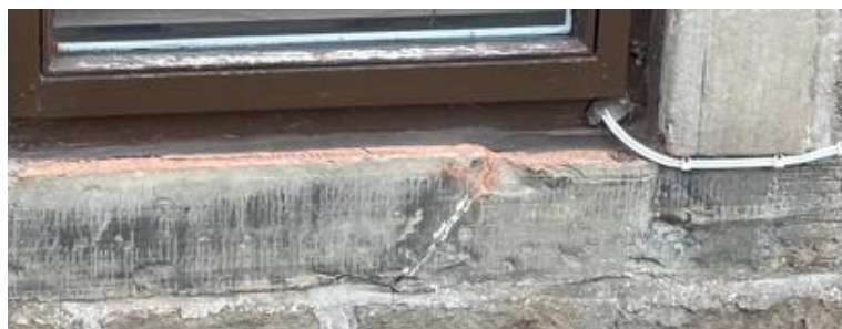
Right, ground floor window to westerly elevation - splitting to right side jamb and cracked cill.
