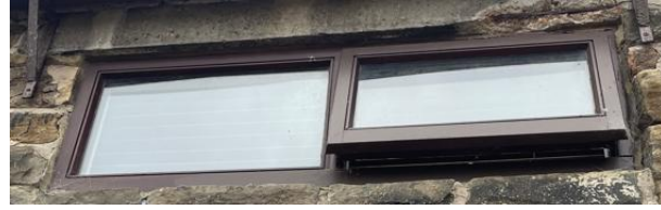
Bedroom Window to Northerly Elevation
