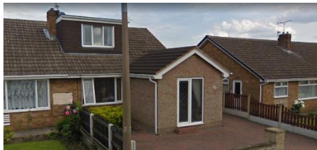
Example of existing dormer with cladding
