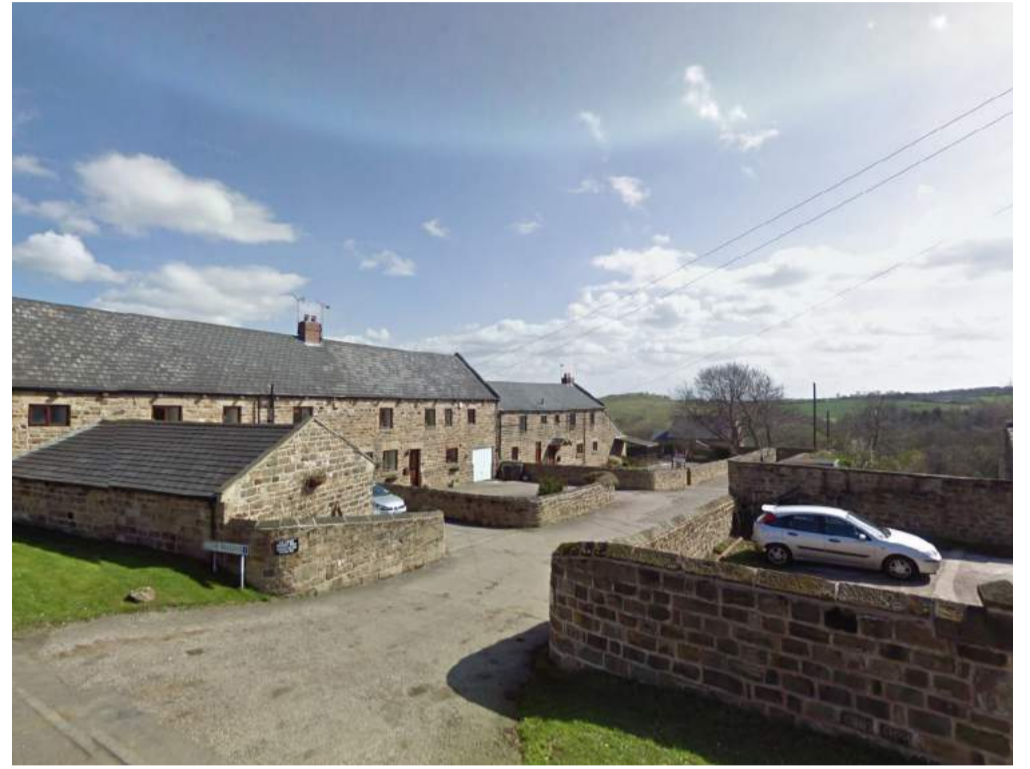
LOCAL AREA VIEW 2: FARM HOUSE ON BEECH HOUSE ROAD
