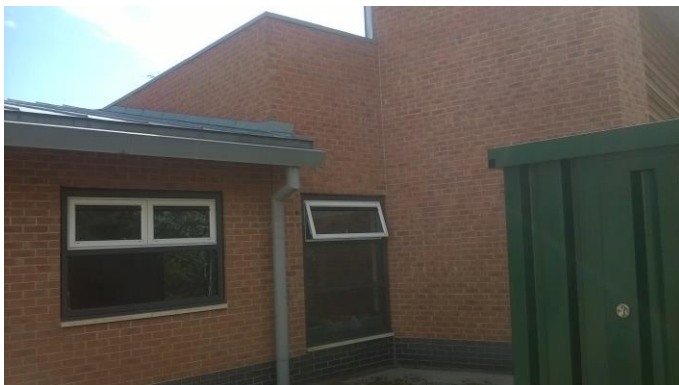
Elevation facing NW and SW
