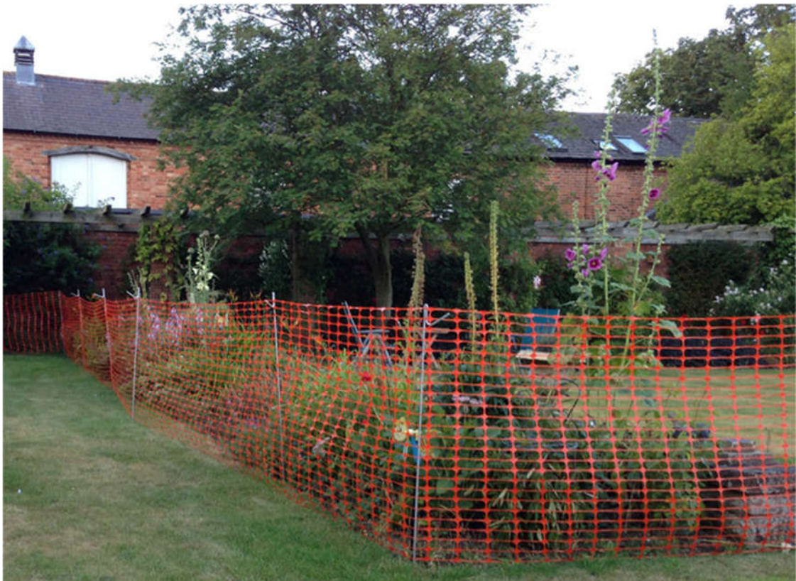
Figure 5: Plastic mesh fencing secured with heavy duty metal stakes
