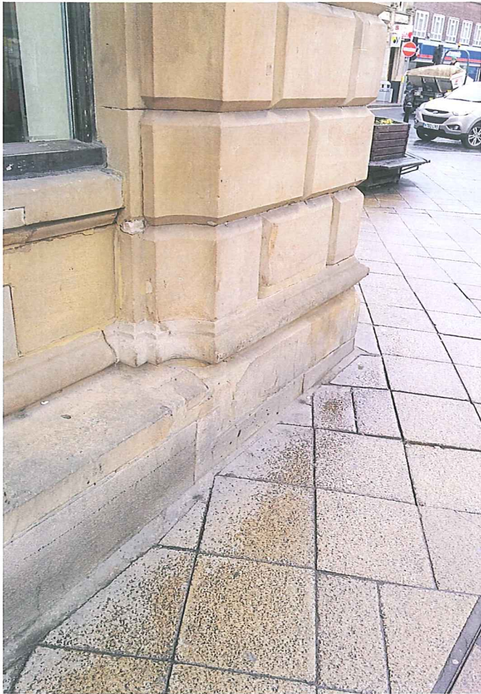
21) LOW LEVEL DETAIL ON PEEL SQUARE ADJACENT ENTRANCE
