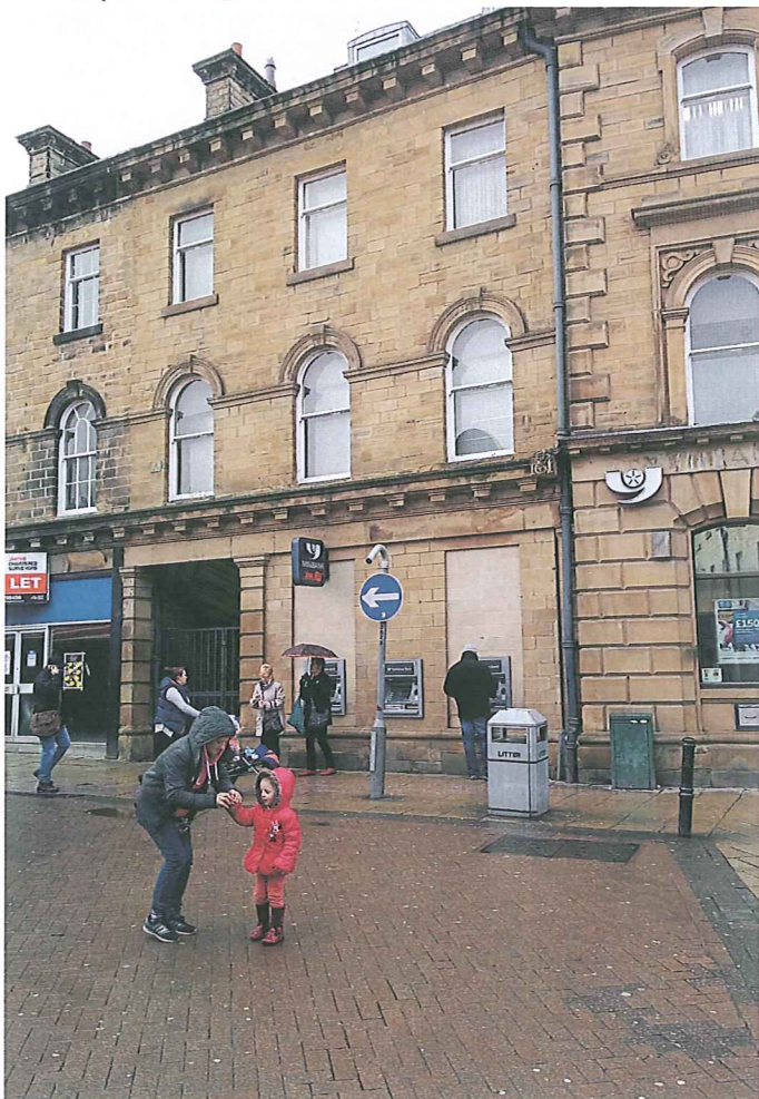
15) EXTENT OF DAMAGE TO PEELE SQ.
