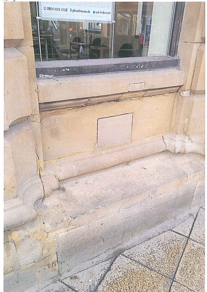
20) WINDOW SILL ADJACENT ENTRANCE TO PEEL SQUARE
