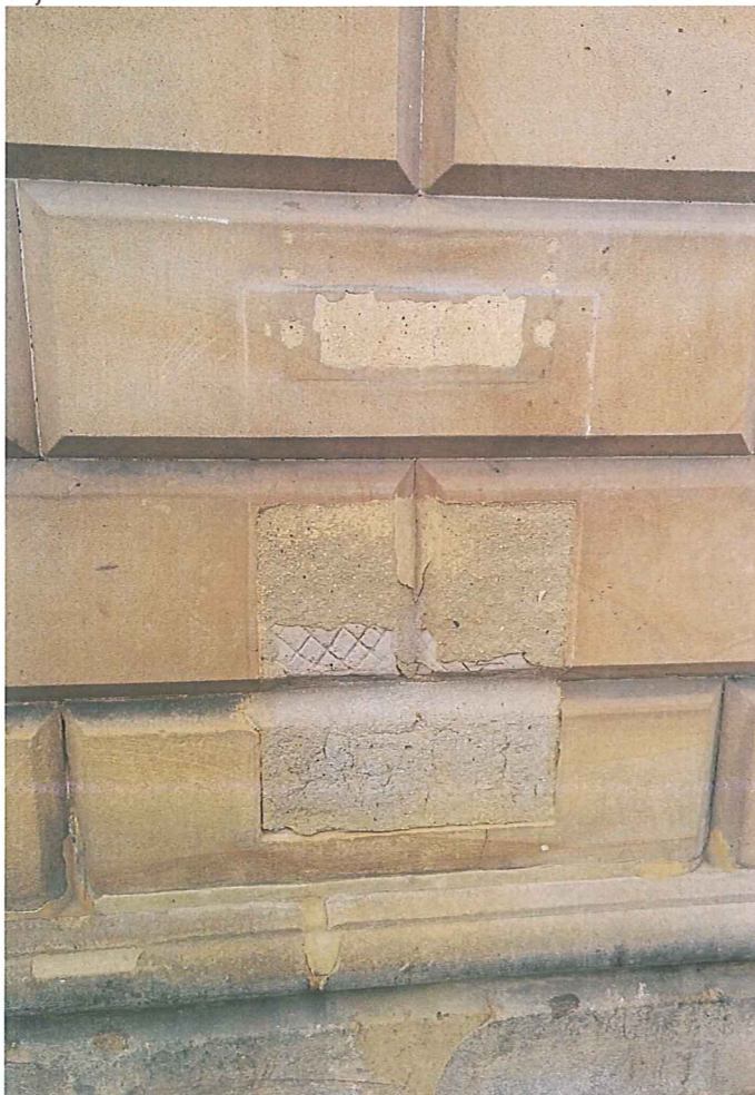
19) EXAMPLE OF PREVIOUS WORK / MAKING GOOD
