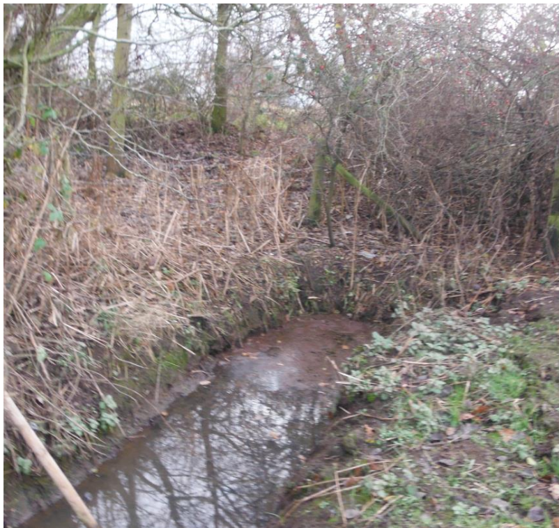
Figure 2-2: Drain discharge through culvert to River Dove
