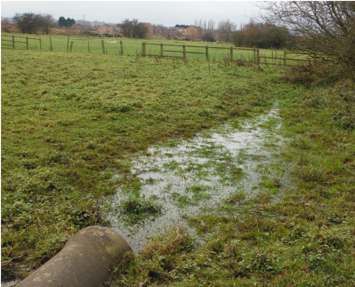
Figure 2-6: Drain Entering the Site from the West
