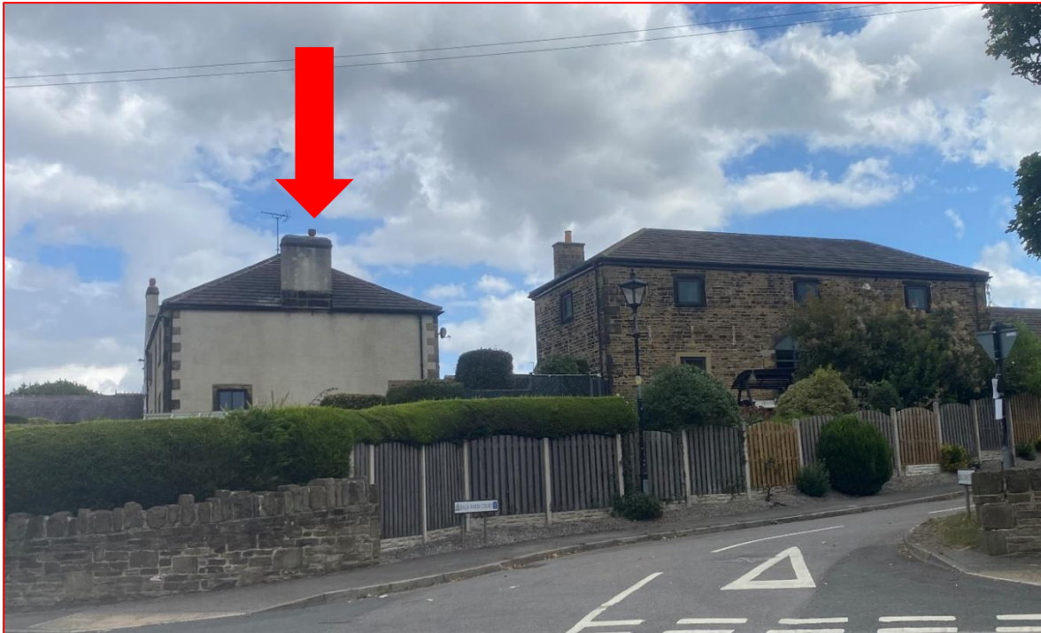
Plate 3: The west elevations of Balk Farmhouse (NHLE 1151049), indicated by red arrow, and the Barn (NHLE 1192453 - right). Note that this view is taken looking east.
