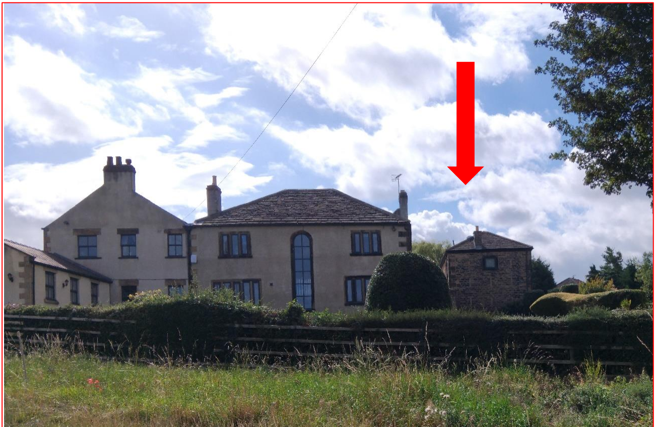
Plate 1: The north facing elevation of Balk Farmhouse (NHLE 1151049 – centre left), and later extensions. The north (side) elevation of the Barn (NHLE 1192453) is indicated by the red arrow. Note that this image is taken looking south.
