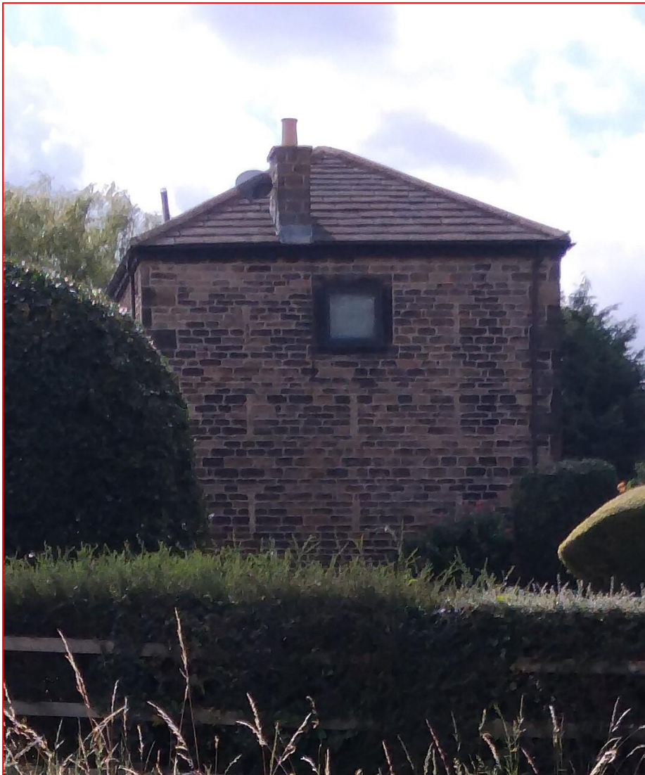
Plate 6: North facing elevation of the Barn (NHLE 1192453). Note that this view is taken looking south and shows the infilled slit window openings and modern high-level window.
