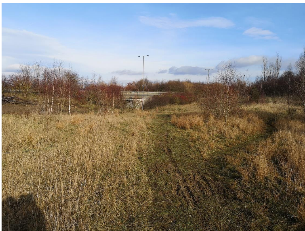
Plate 3: View to the underpass on the A6195 at the north-eastern corner of the site
