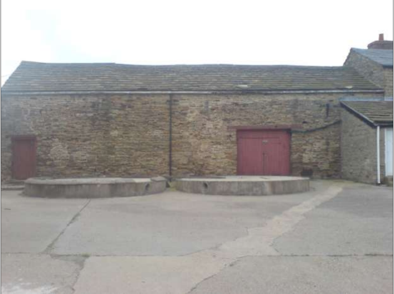
Photo 2: Old silo foundations.
