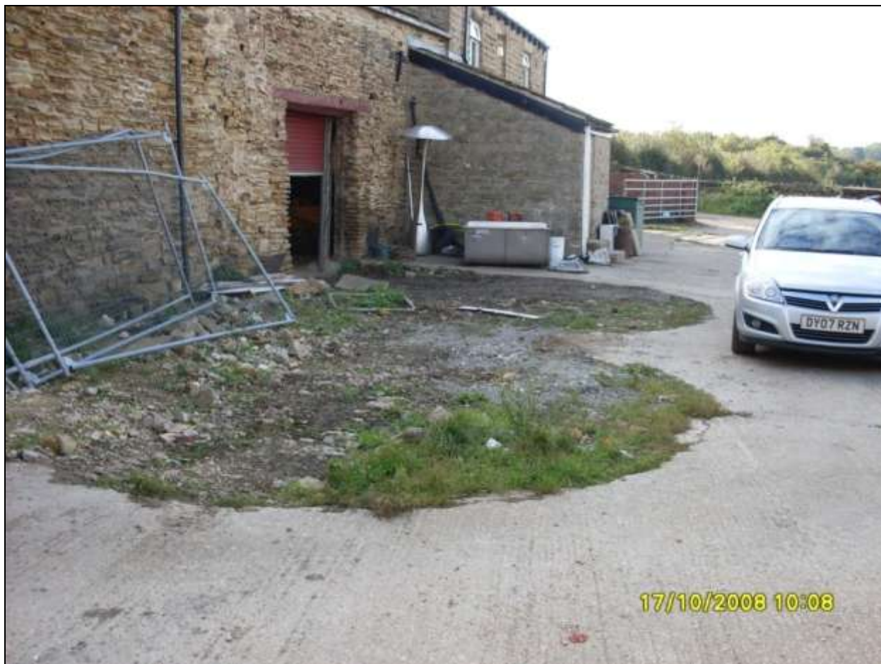
Photo 3: Removed silo foundations (looking south)
