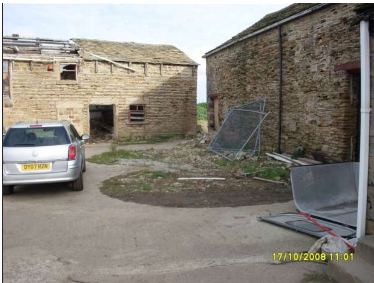
Photo 4: Removed silo foundation (looking north)
