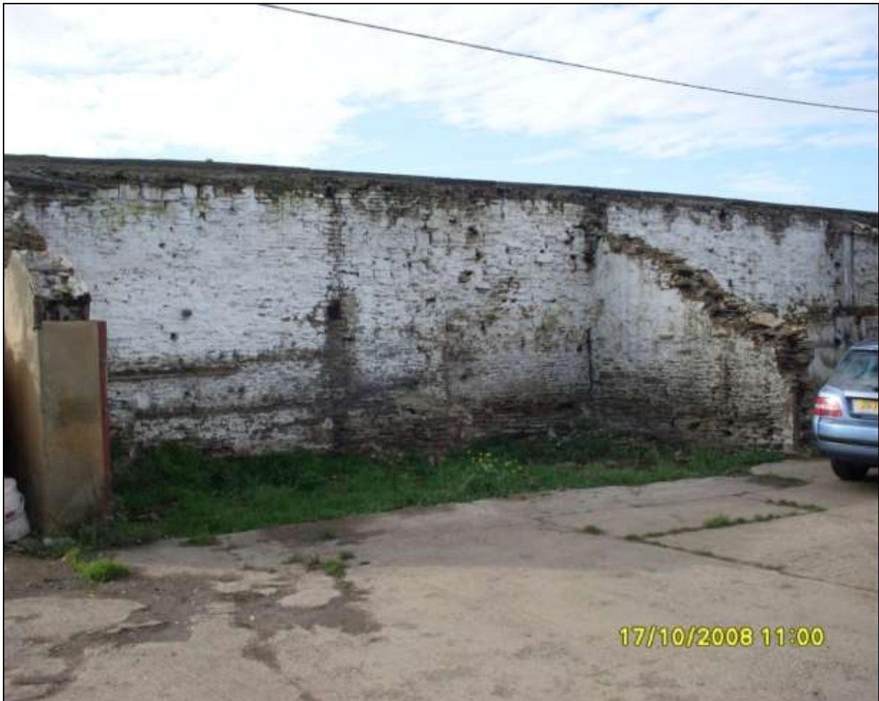
Photo 1: Partially demolished barns, south of the courtyard
