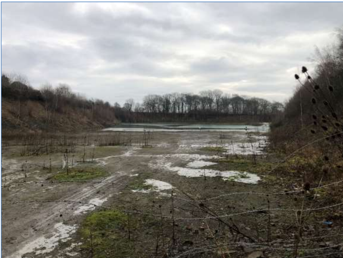
Plate 4: View southeast across the Site from the entrance at the southwest corner
