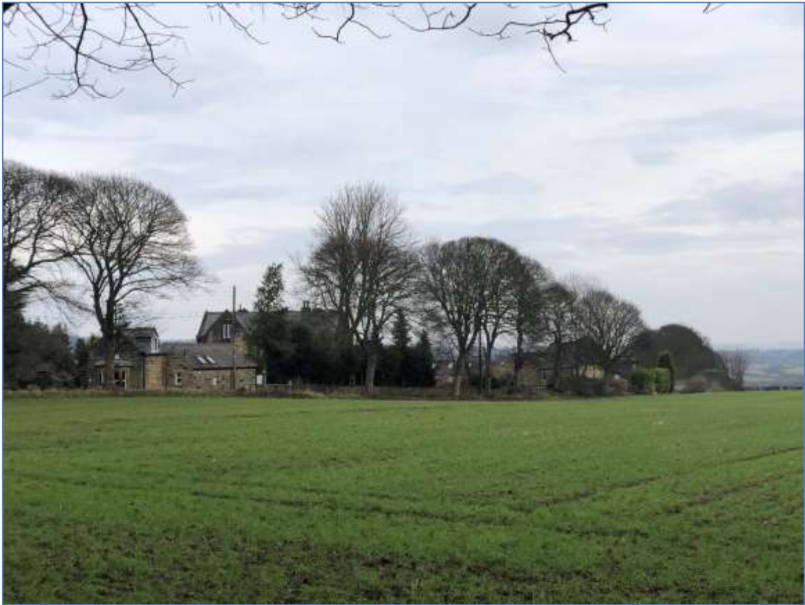
Plate 11: View east towards the Swaithe Listed Buildings (Assets 1, 2, and 6)
