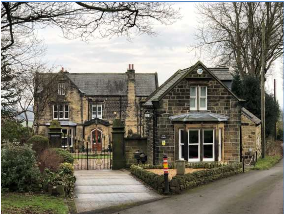
Plate 12: View east of Swaithe Hall and Farmhouse (Asset 1)
