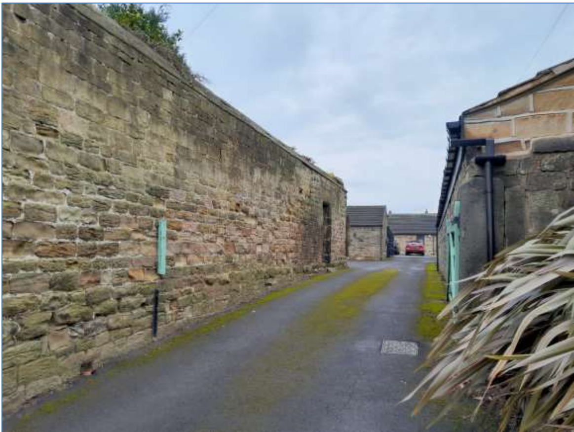
Plate 16: View north of entrance to Ardsely Manor House (Asset 3) and Cartshed (Asset 9) on Doncaster Road
