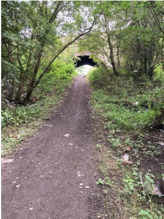
Figure 3: Image, looking south, of the A61 highway bridge arch infill and formed incline.
