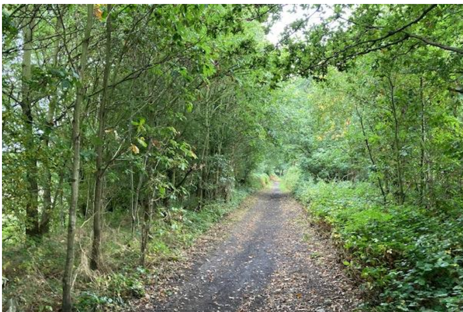
Figure 6: View of the route on top of the raised embankment, looking south.
