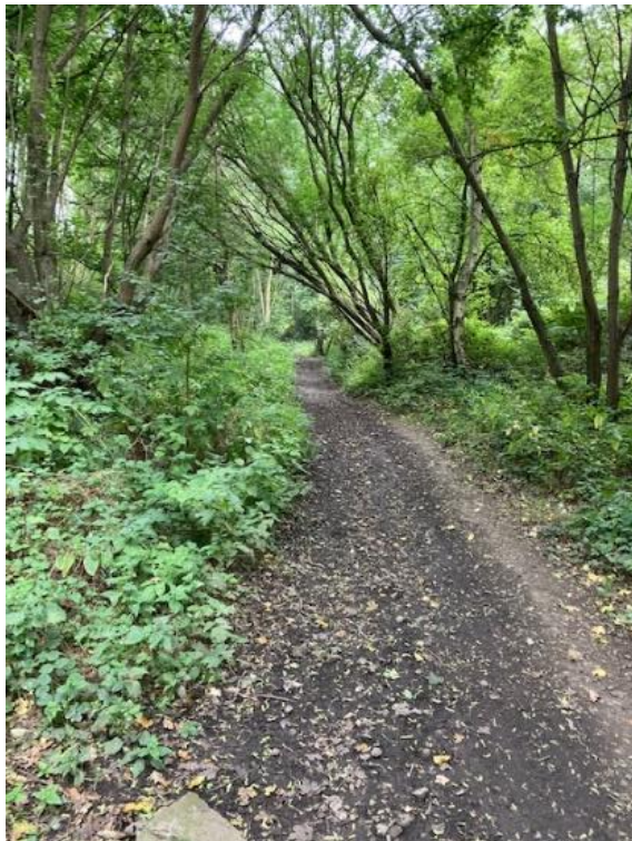
Figure 4: View looking north within the cutting.
