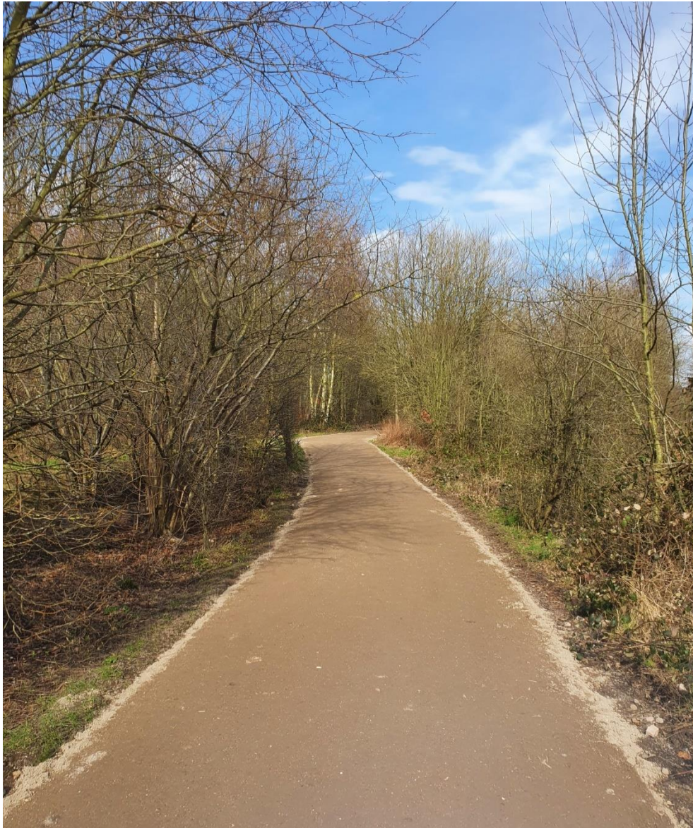
Figure 7: Bridleway construction example on the TPT at Elsecar, surfaced with 6mm to dust aggregate.
