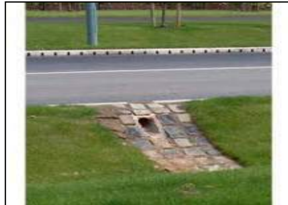
Photo showing gully into swale
