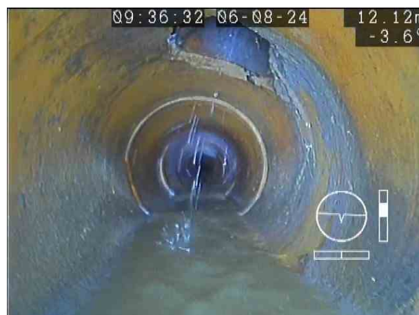
MH1X_c03737ab-b56c-44e3-8d3f-9695d96e3ca8_20240812_111333_891.jpg, 00:01:13, 12.12 m Connection other than junction at 01 o'clock, 100mm dia
