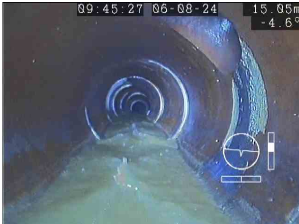
MH2X_a38a3649-f45a-43d8-9154-86ef85ffa054_20240812_111802_344.jpg, 00:01:35, 15.05 m Junction at 01 o'clock, 100mm dia
