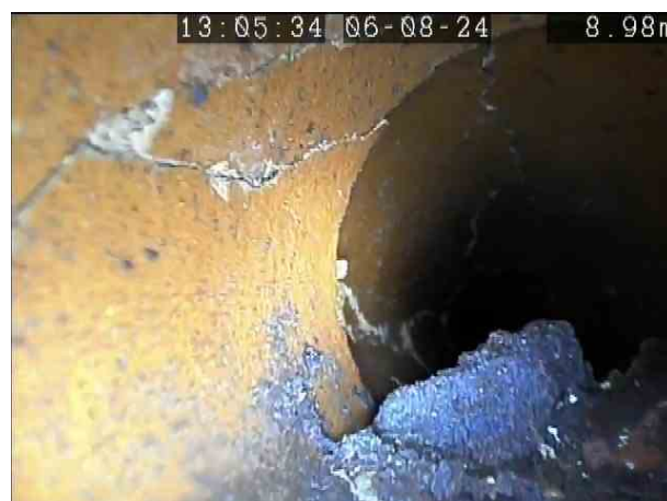
MH4X_7d501f97-82de-4354-9a49-4944b60663d8_20240812_120423_882.jpg, 00:00:51, 8.98 m Settled deposits, fine, 30% cross-sectional area loss
