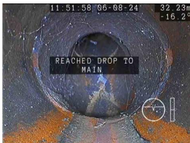
Exc Pipe1X_6996a05f-2b40-46db-a197-b5ac073126dd_20240812_113859_811.jpg, 00:03:19, 32.23 m Finish node, other special chamber, reference: Downstream, Reached drop to main
