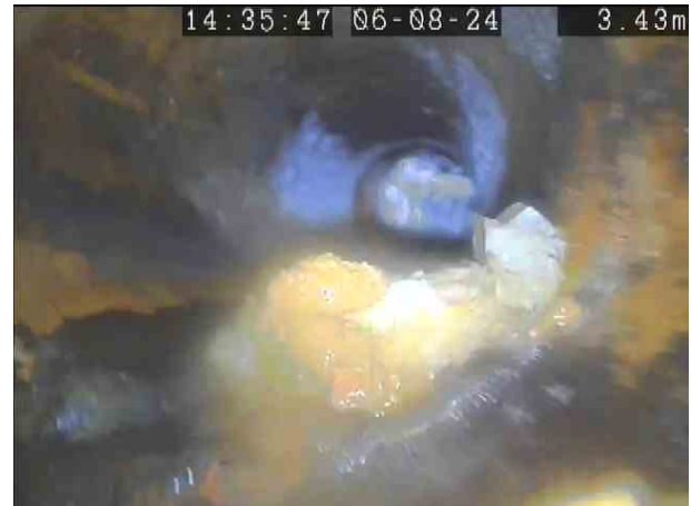
MH9X_549ea207-83ad-44cc-b032-0152d315ed48_20240812_121140_525.jpg, 00:00:24, 3.43 m Attached deposits, fouling from 04 o'clock to 07 o'clock, 15% cross-sectional area loss
