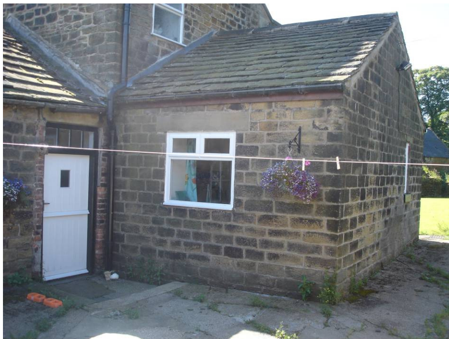
02. Courtyard view of North Elevation and entrance door.
