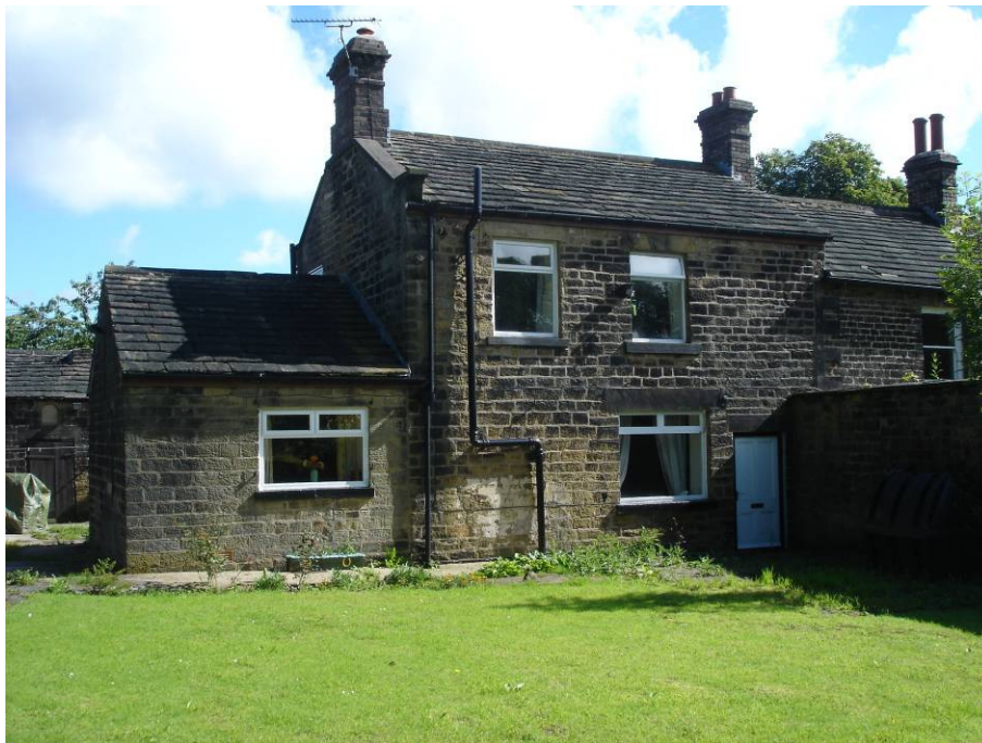
Carlton House Cottage – South Elevation
