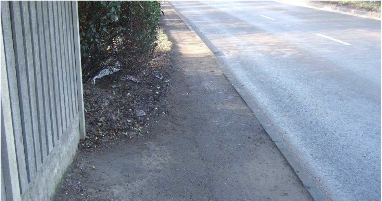
Figure 3 Shaw Lane footway narrowing to 700mm wide west of the proposed toucan crossing
