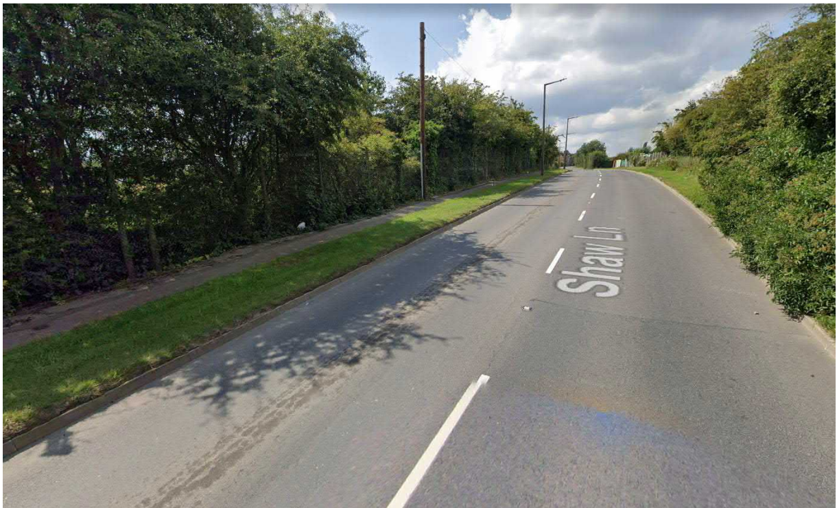
Figure 4-1 Existing Footway on Shaw Lane (Source: GOOGLE)
