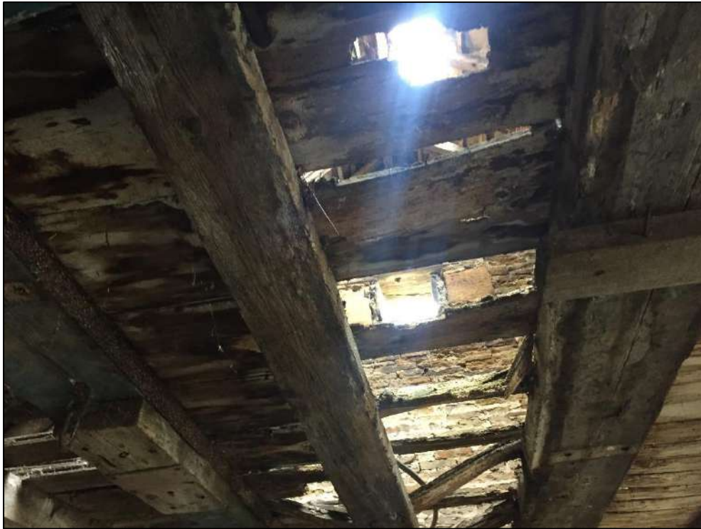
Plate 17: Detail of ceiling in building 2
