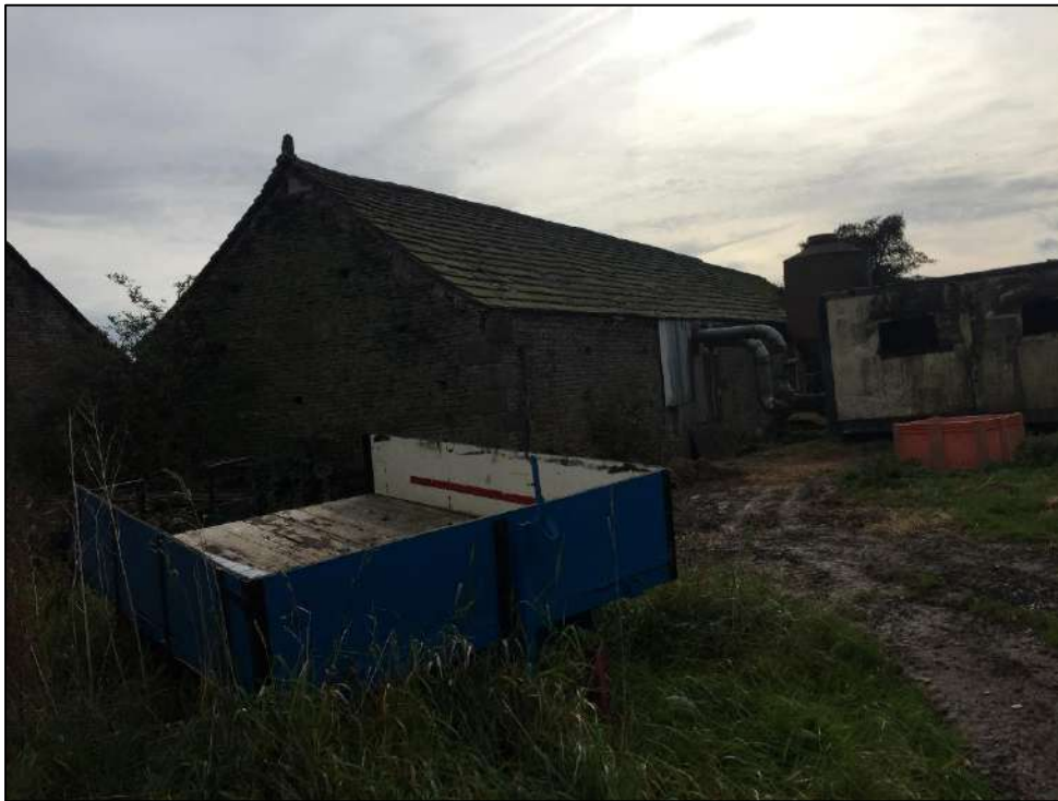
Plate 3: West aspect of building 1
