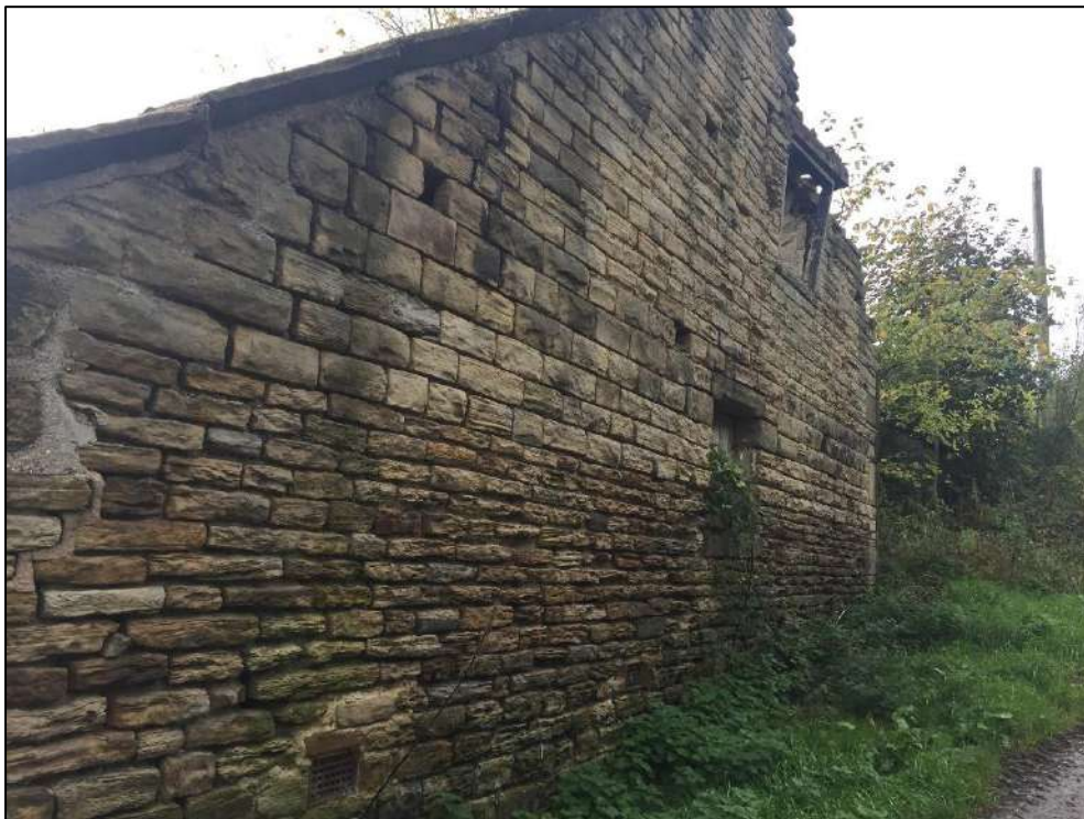
Plate 20: North aspect of building 3
