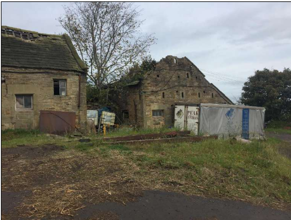
Plate 18: South aspect of building 3
