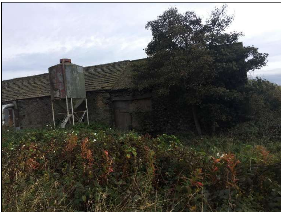
Plate 4: West aspect of building 1
