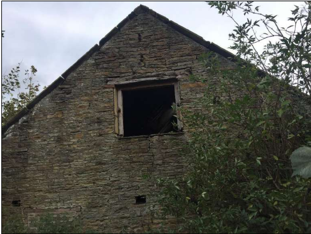
Plate 15: West aspect of building 2
