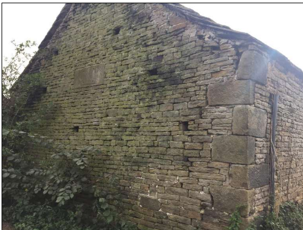
Plate 14: Northwest aspect of building 2
