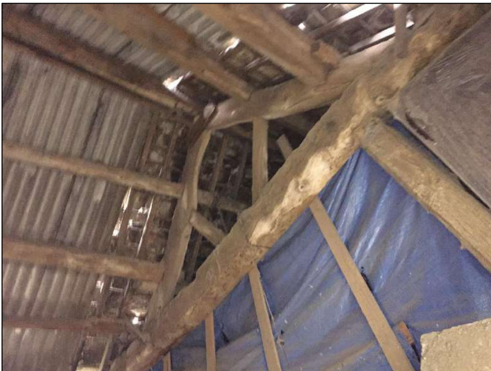
Plate 10: Detail of interior roof of building 1
