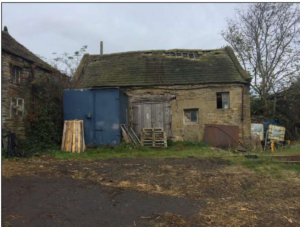
Plate 13: South aspect of building 2
