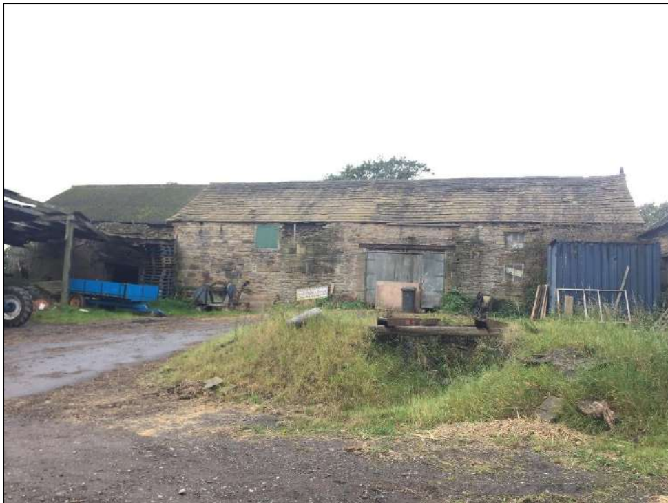
Plate 6: East aspect of building 1 and adjacent hard standing and ephemeral vegetation
