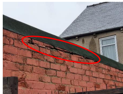
Outbuilding - damaged brickwork
