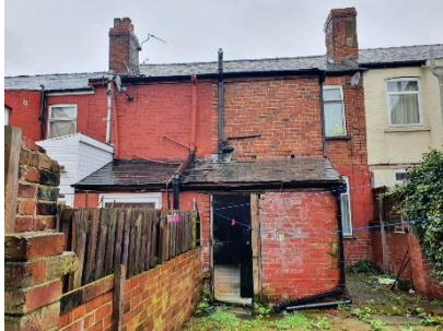
Housing - broken and slipped tiles
