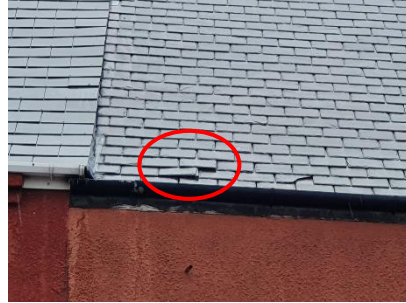
Housing - lifted flashing
