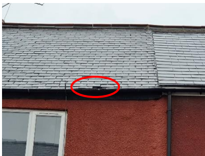
Housing - broken and slipped tiles
