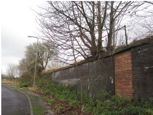
Plate 3.3: View of brick wall in good condition
