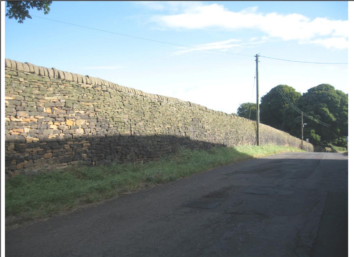
Photo 1: Existing stone boundary wall on Chapel Lane
