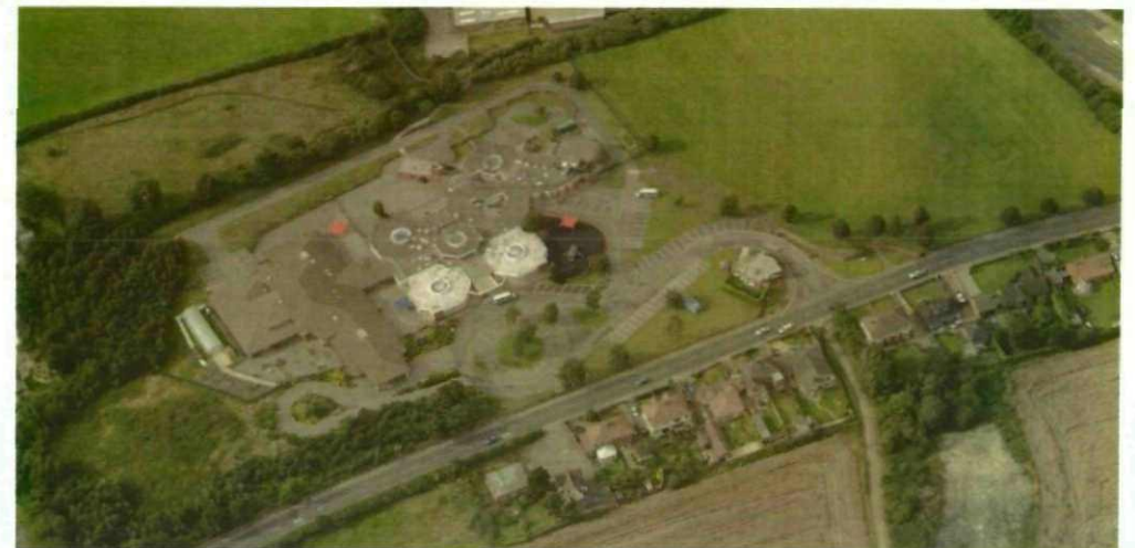
Fig. 7 Site aerial photo from South West
