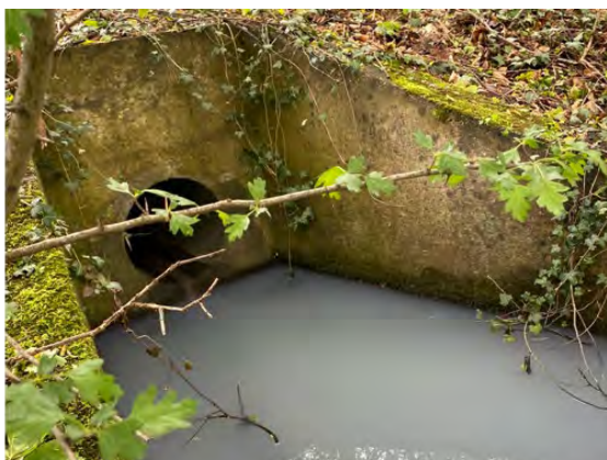
Photo 5: View of small 300mm culvert discharging into unnamed stream adjacent the culvert
