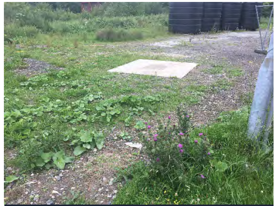
Photo 8: View of drainage inspection cover on eastern plot
