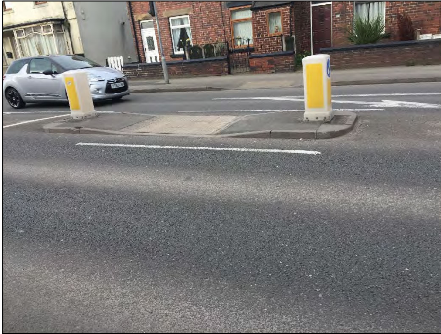
Image 2.5 Pedestrian Refuge Island on Sheffield Road
