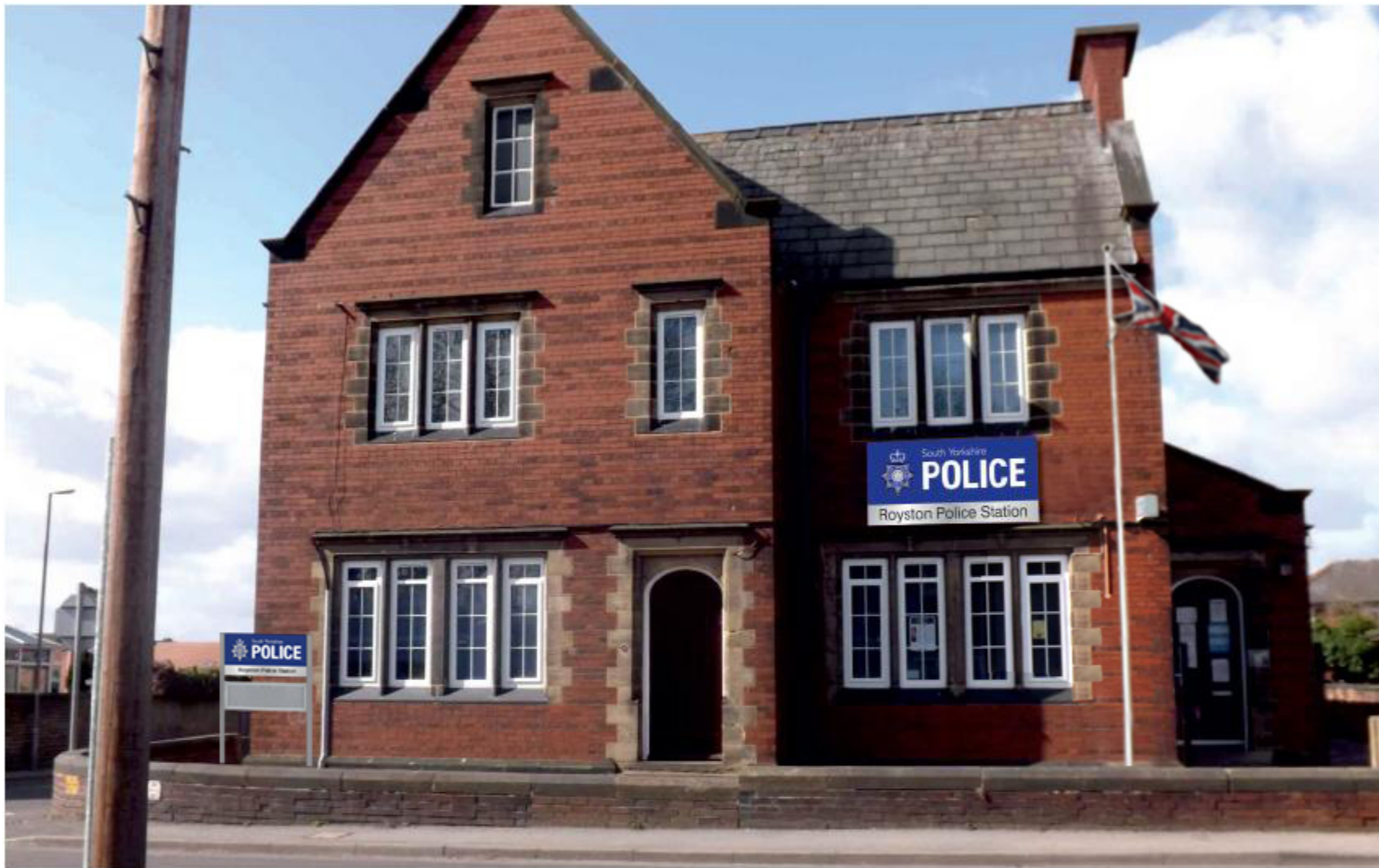
Front elevation Royston Police Station, Barnsley
