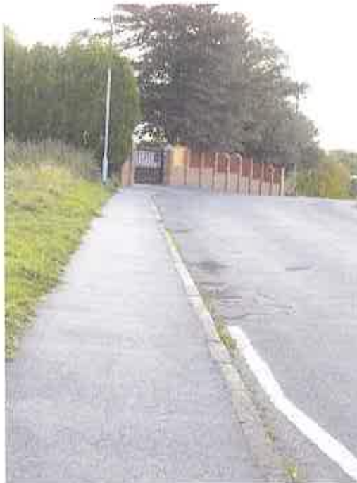
Plate 6 – Typical footway on Burntwood Road
