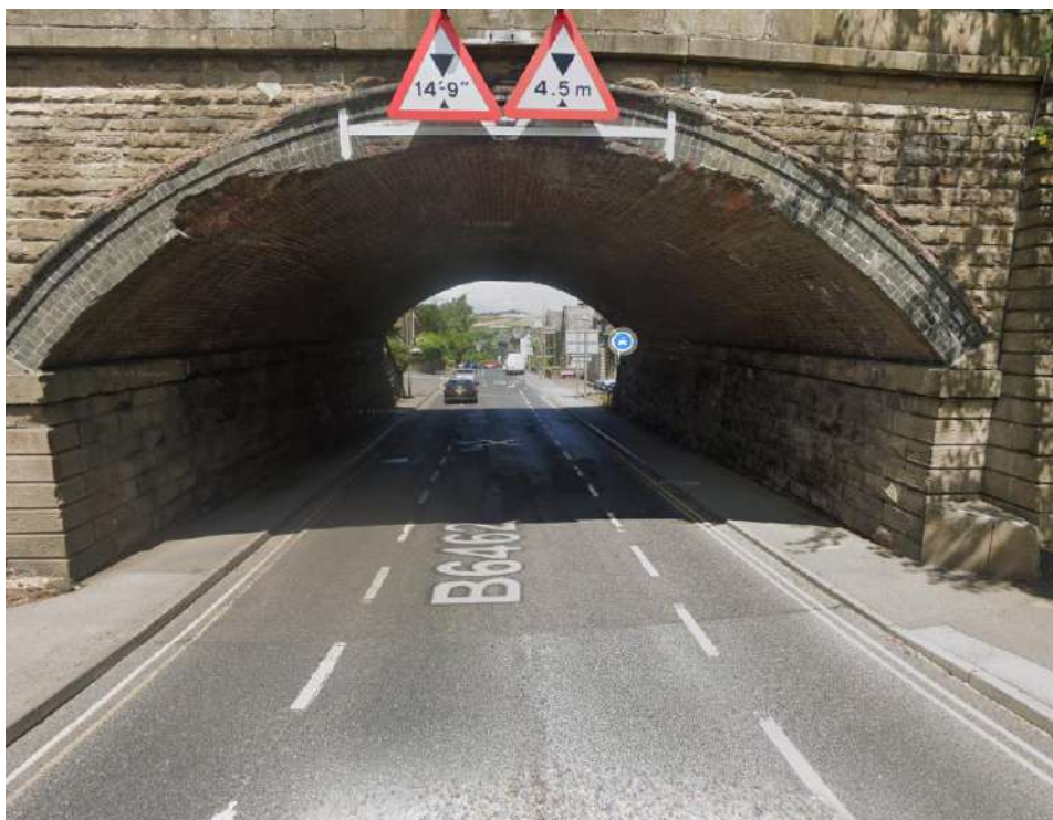
Figure 5 – B6462 Bridge Street northbound
