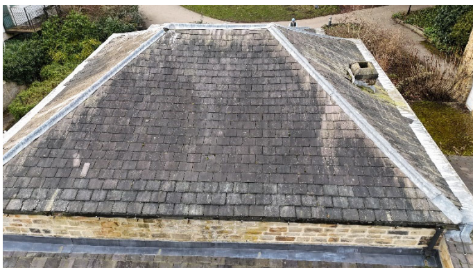
East facing roof pitch
