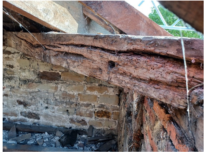
Flight holes in the dragon beam tie to the southeast corner
