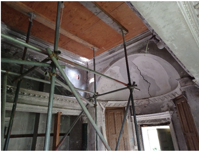
View of ceiling and supporting scaffold structure in G1
