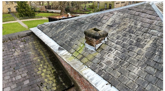
North facing roof pitch
