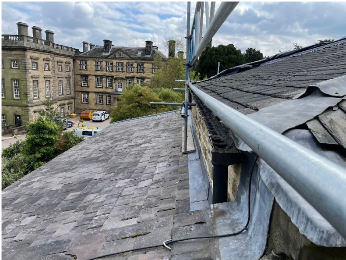
View of the gutter from the north side
