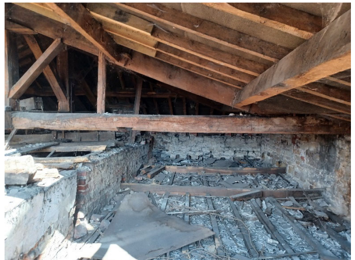
View of the ceiling structure to the upper ceiling in G2
