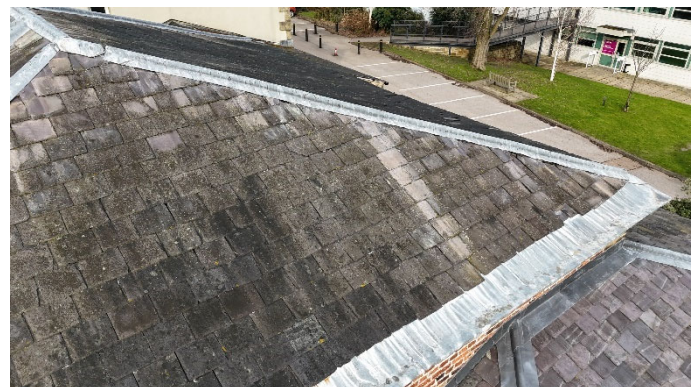
South facing roof pitch
