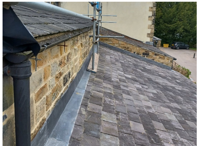
View of gutter from the south side
