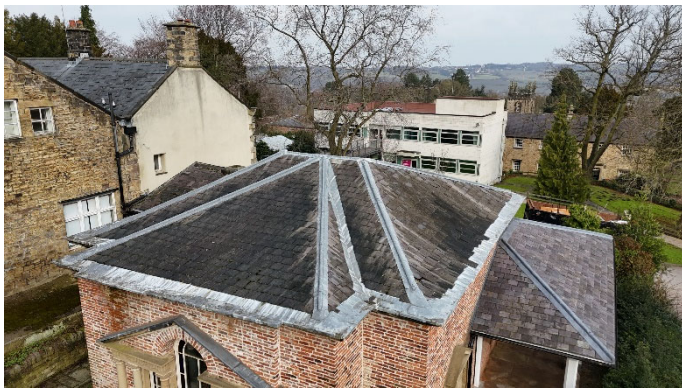
West facing roof pitch
