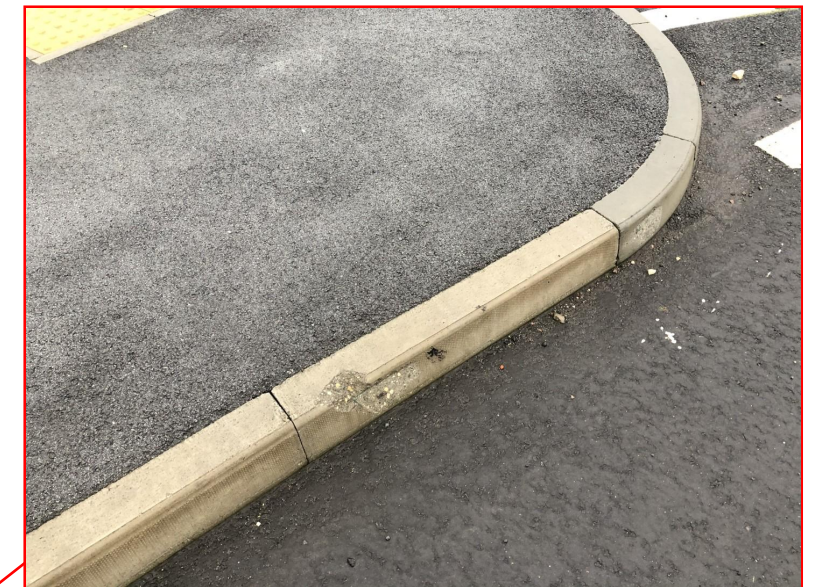
Chipped kerb on splitter island.
