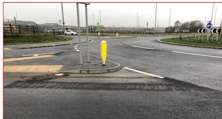
Existing road markings are in the process of being burnt off and repainted, extent of these works is unknown.
