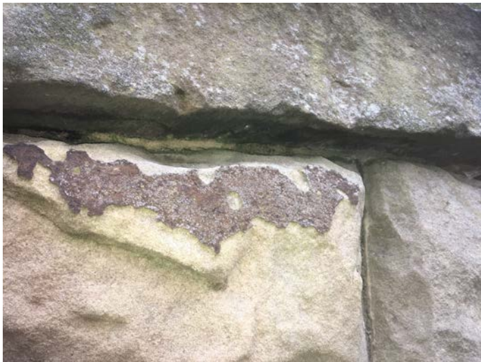
Bridge mortar detail
