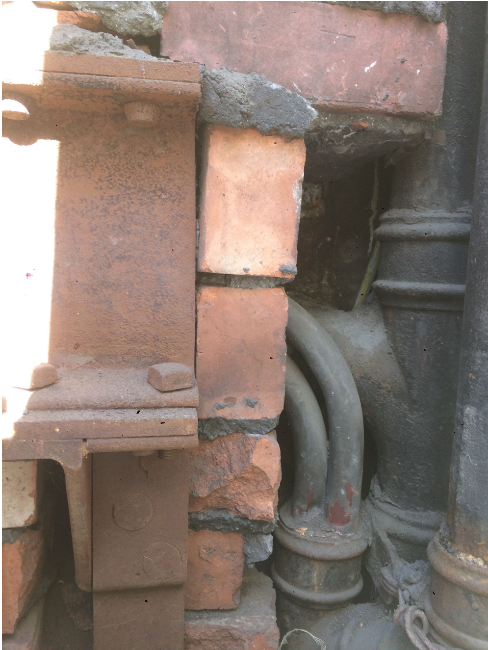
Right-hand end of bressumer beam
