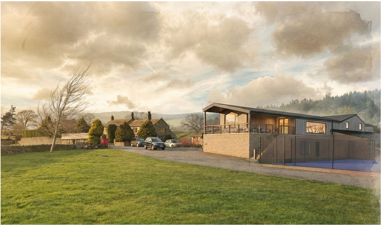
Contextual visualisation showing listed building in the background
