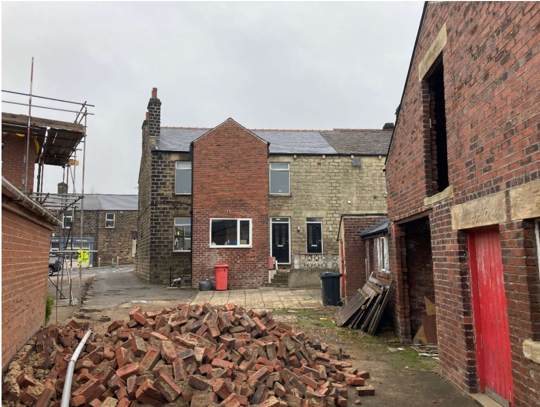
Fig 05. View of rear of 2 Blacker Road from the site of the prop extension looking north.
