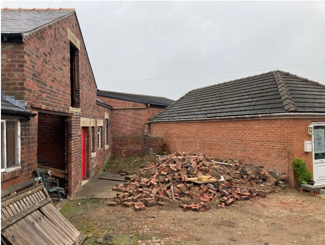
Fig 03. View of site for single storey extension looking south.
