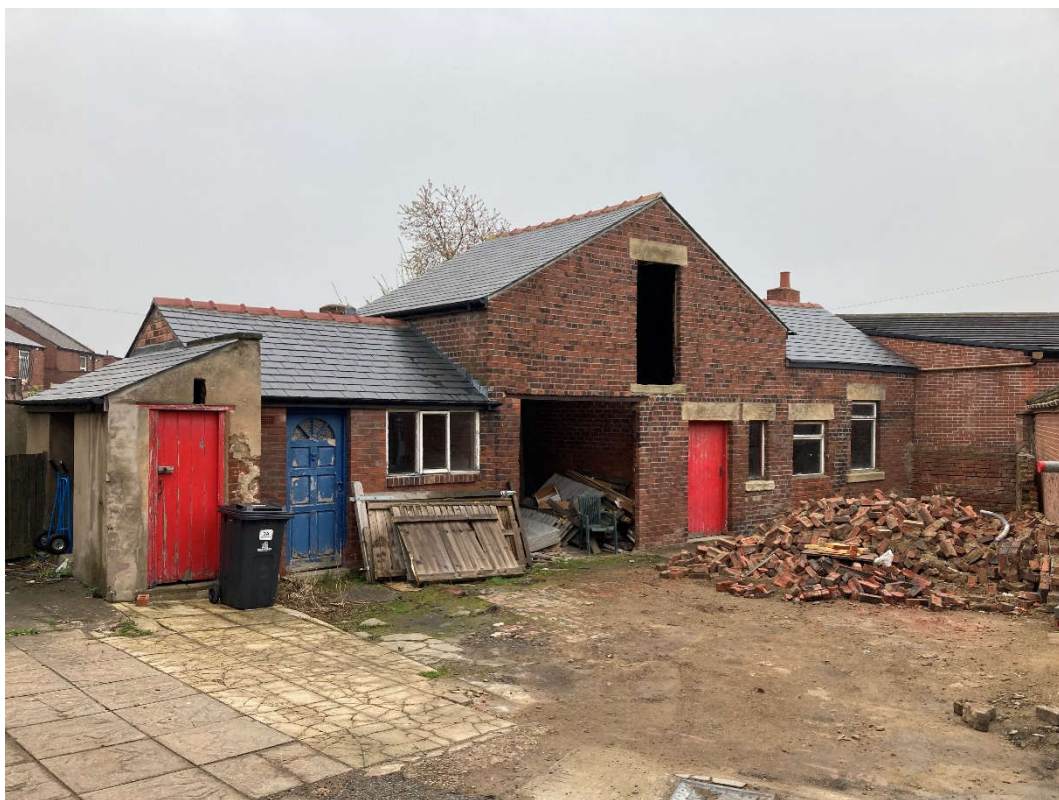
Fig 02. View of existing Outbuildings looking east.
