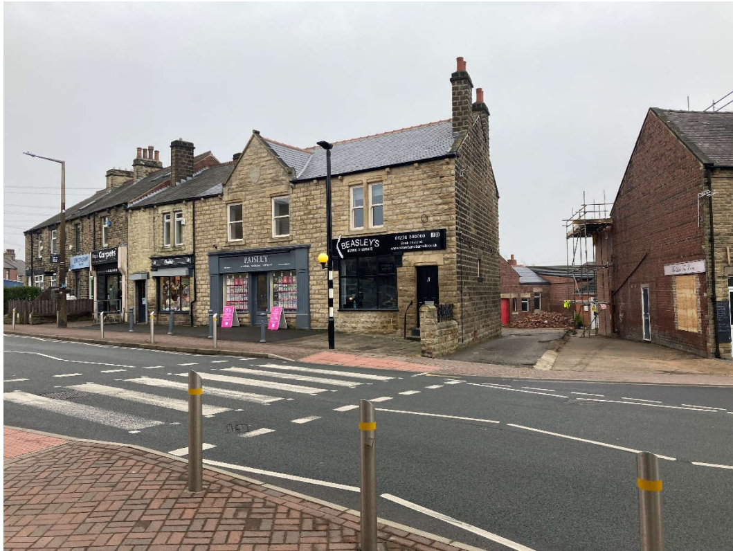
Fig 01. View of access from Blacker road looking south east.
