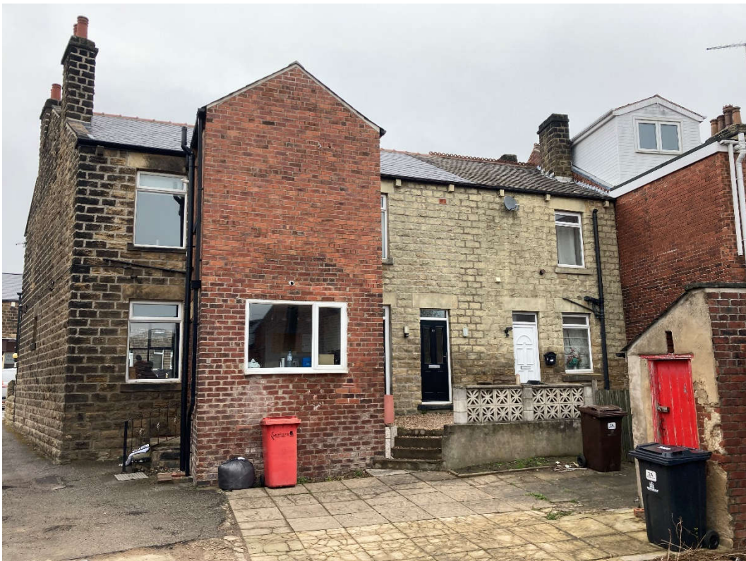
Fig 05. View of rear of 2 and 4 Blacker Road looking north.
