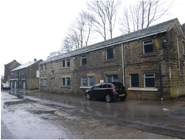
Existing unused offices to be demolished – North west view
