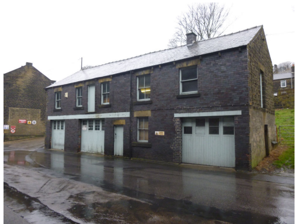
Existing Office building to be demolished – North view
