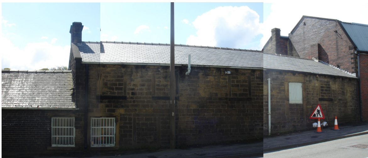
Image of existing offices to be refurbished into residential apartments. South facing view from Manchester Road
