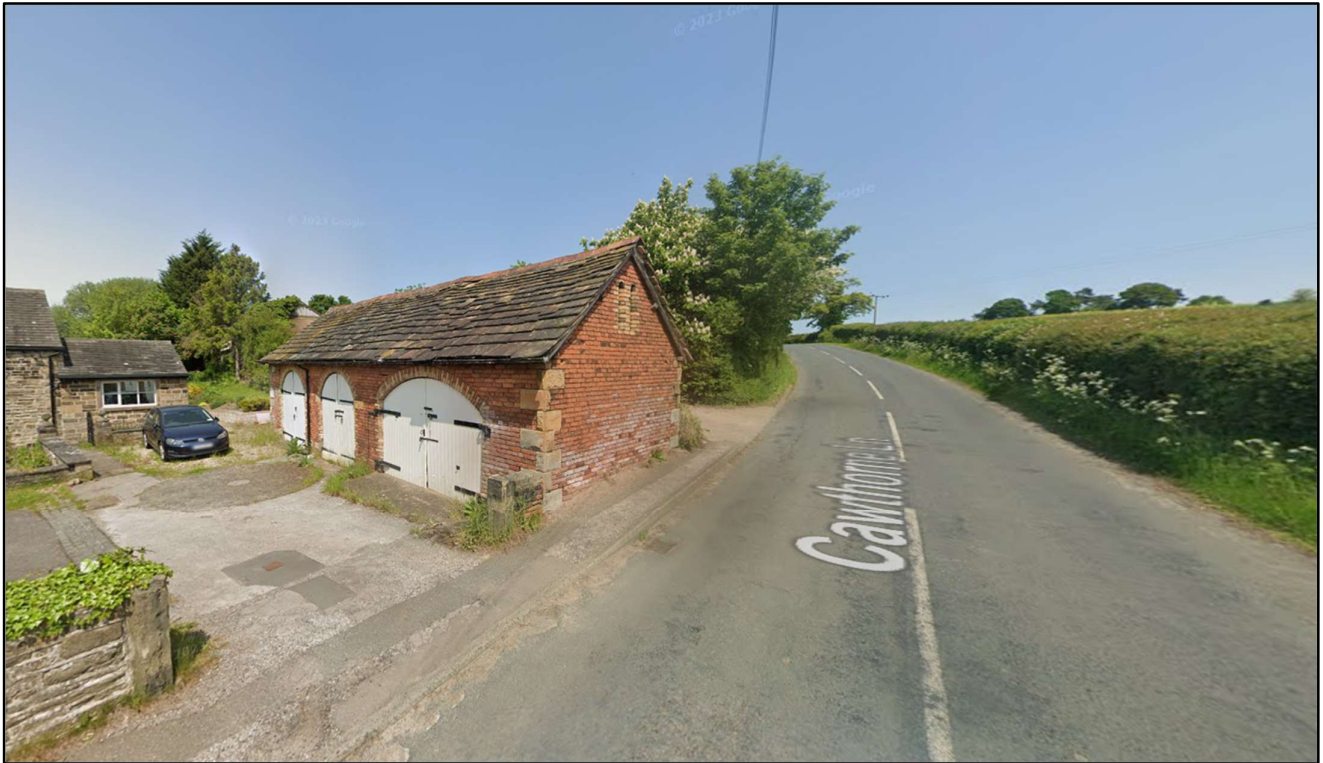
Figure 3 – Photo showing the building to be demolished and the existing access into the site, as well as the view up towards Cawthorne Lane
