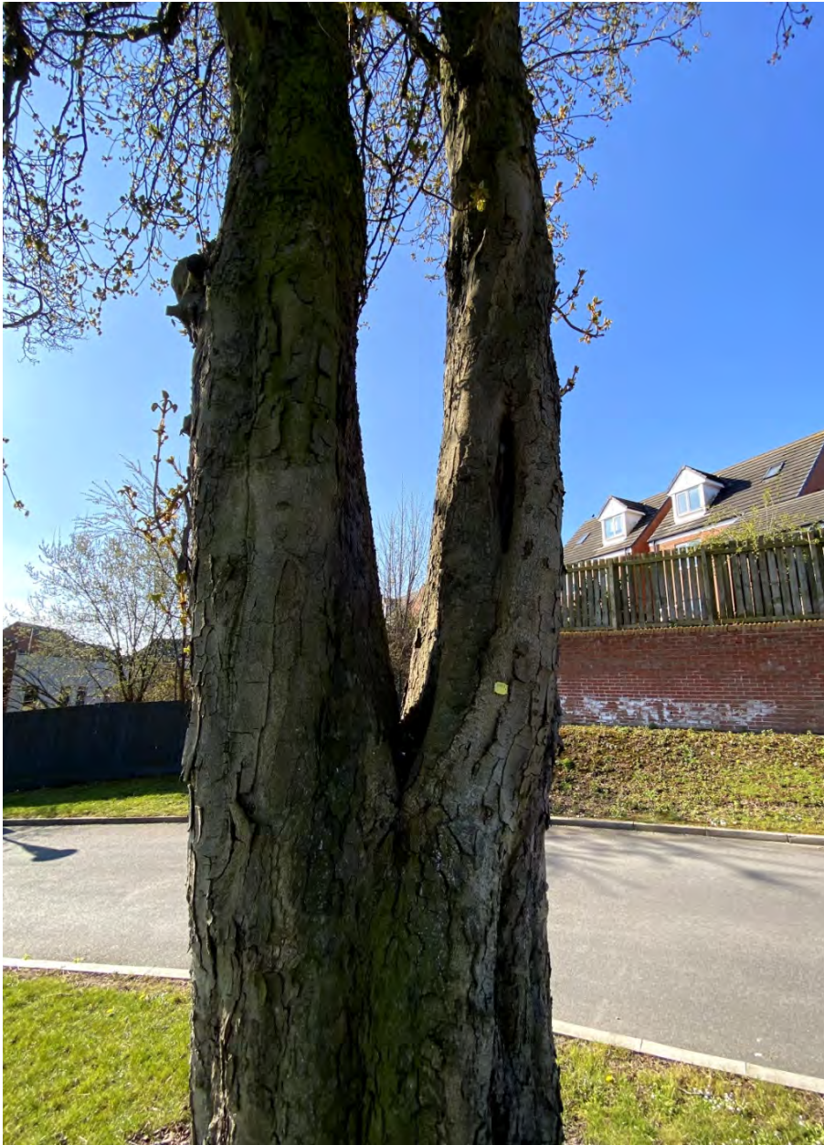
Photographic plate showing the tree 1833 with mechanical damage in the Lower stem..
