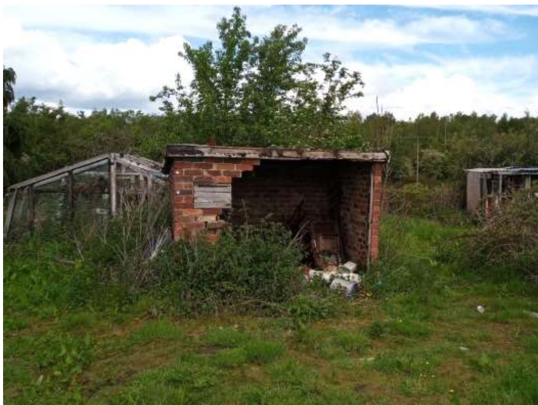
Plate 15: Remains of former allotment buildings
