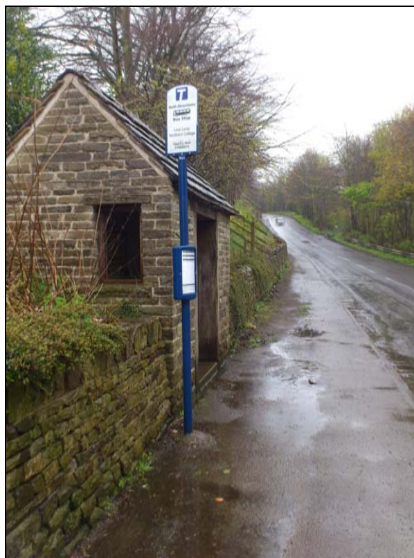
Figure 4.7: Bus Stop on Lowe Lane
