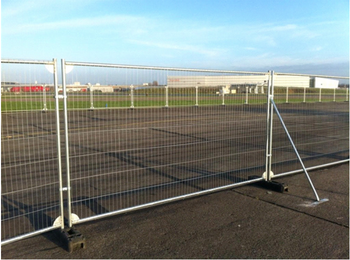
Heras tree protection fencing
