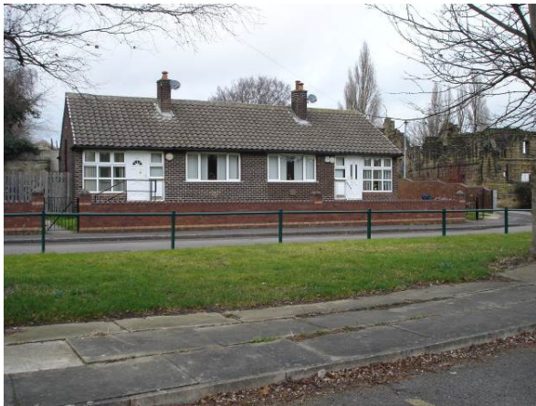
Fig 01. Bungalows on Abbey La to south of site
