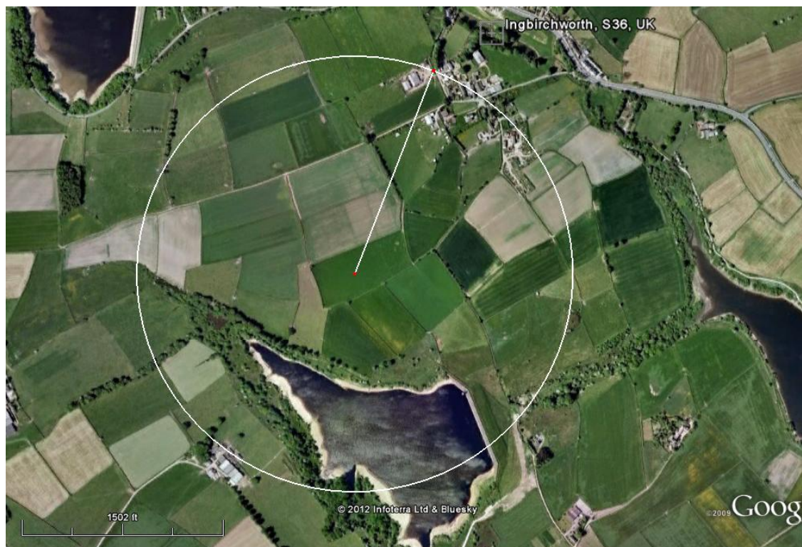
Figure 2: Aerial Photo – Wider Area (Reproduced under licence from Google Earth Pro)
