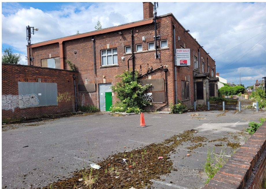
Area to east of hotel building
