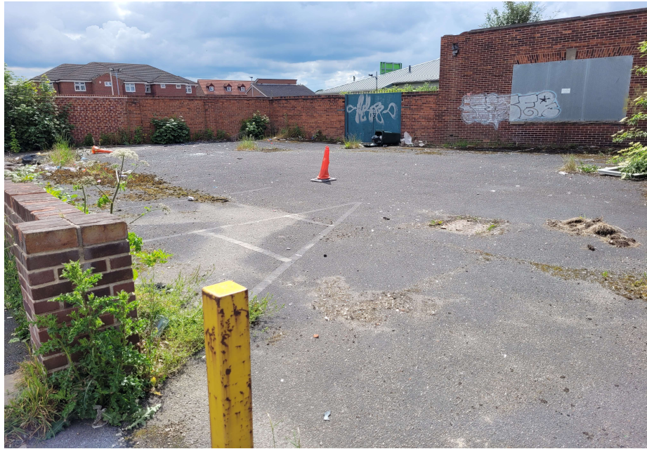
Area to east of hotel building
