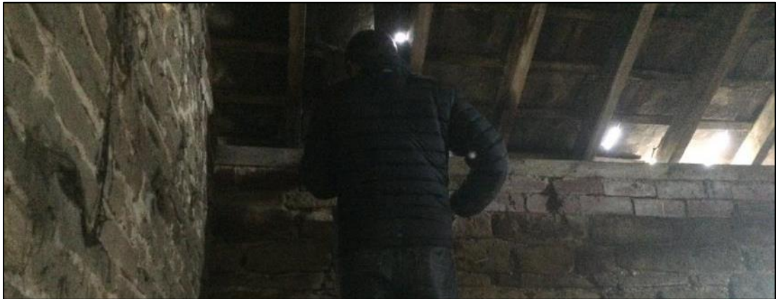
Plate 6. Inspection of wall top from ladder
