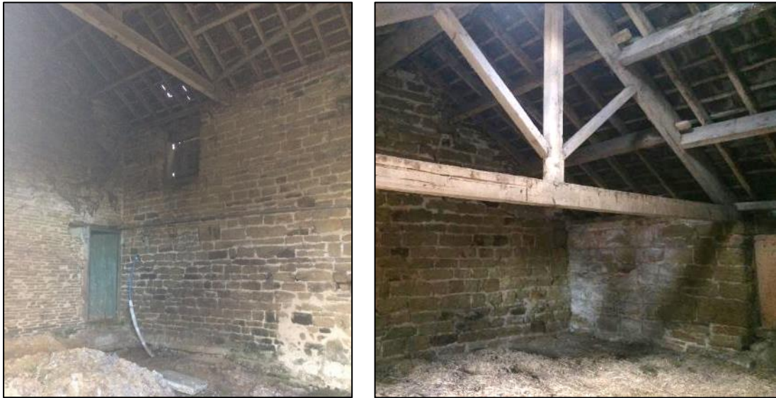
Plate 4. Inside of central section of Building 1 and a first floor compartment within the same building
