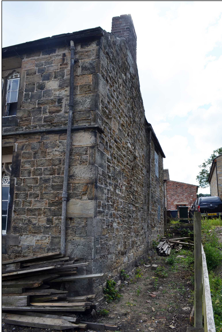
Figure 1: North-west elevation of Bank House
