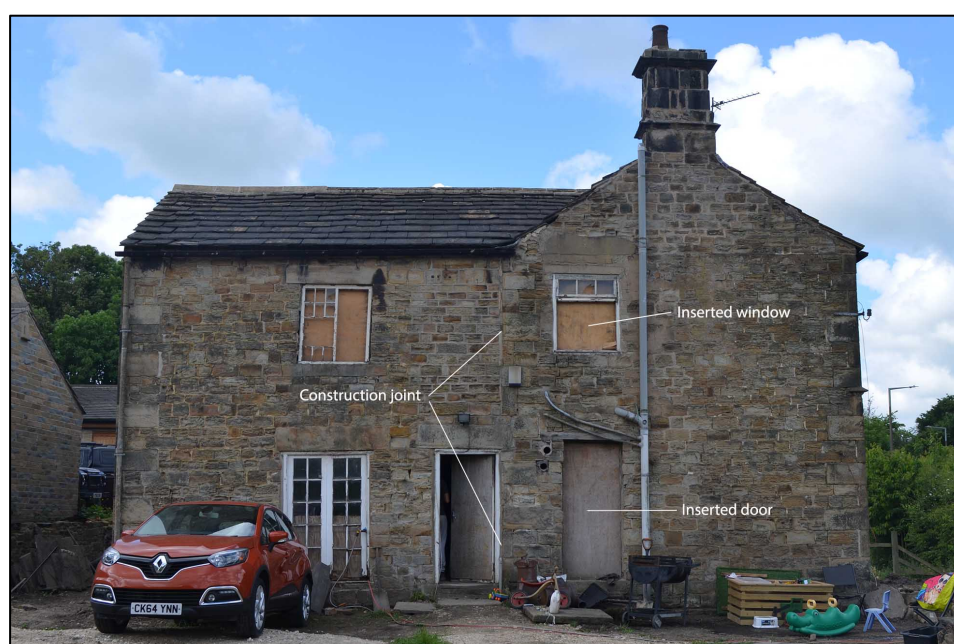
Figure 2: South-east elevation of Bank House
