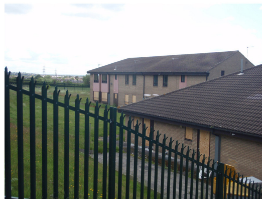
LOOKING SOUTH FROM EMBANKMENT
