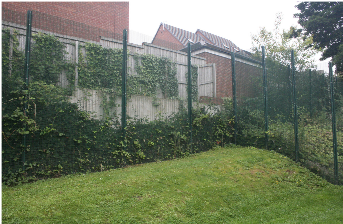
Appendix Fig: 8 - Existing perimeter fencing
