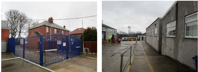
Fig 3; Buildings owned by Balmoral Group either side of site access.
