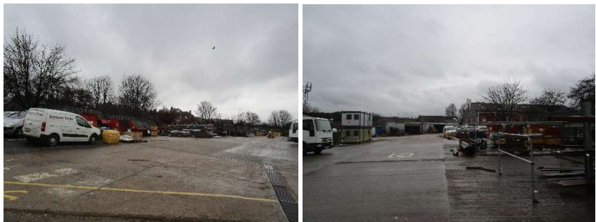
Fig 5; Buildings and areas of hardstanding within the site.
