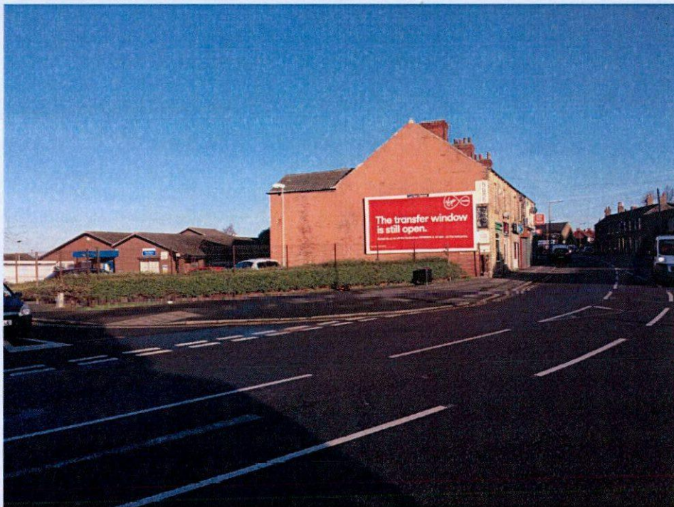
Figure 3. Photograph of the application site.
