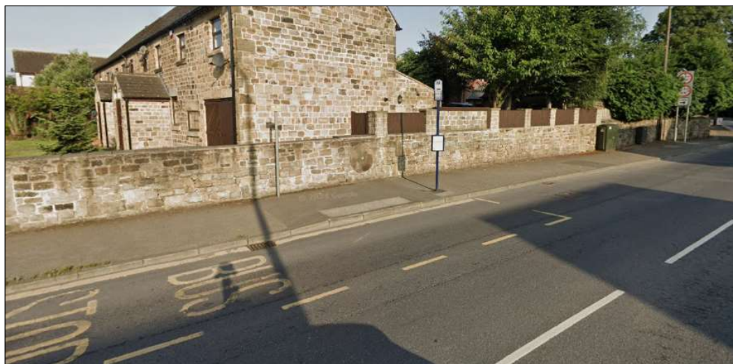
Figure 2. Bus stop 51107 (Fish Dam Lane/Manor Farm Close)
