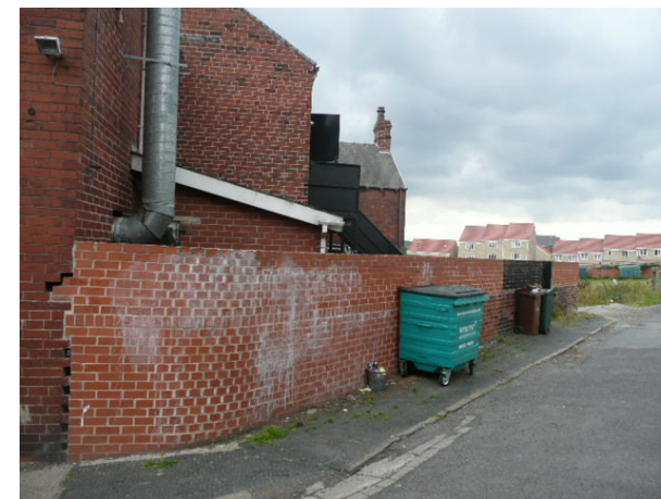
VIEW TO REAR OF 92 TO 98 SNAPE ROAD
