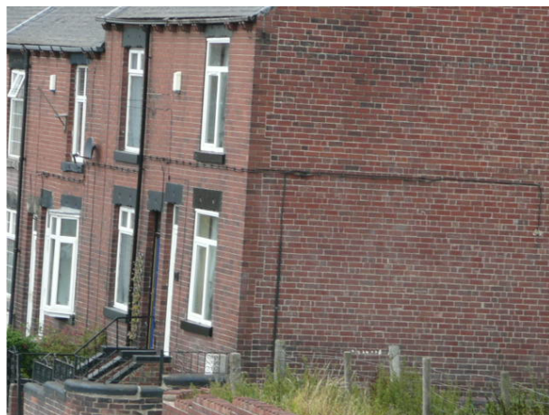
SNAPEHILL ROAD FRONTAGE
