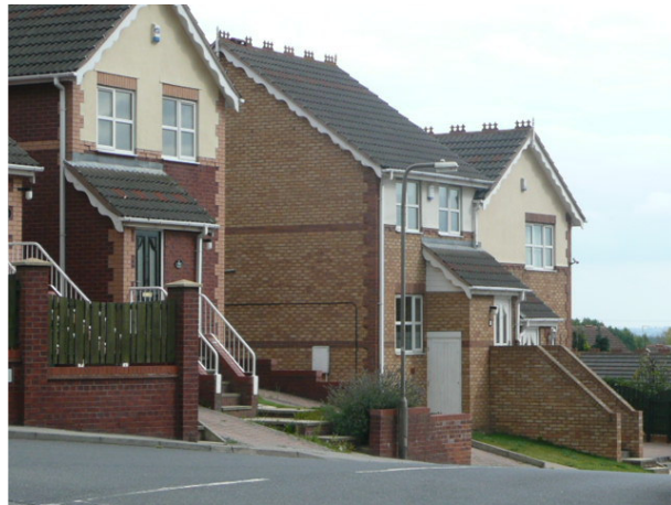
EXISTING HOUSES ADJACENT SITE
