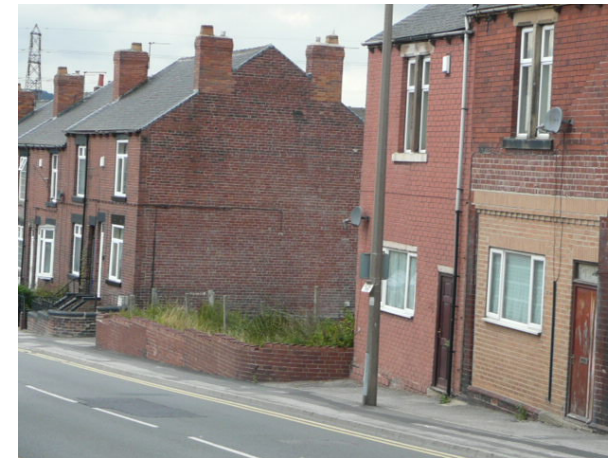
SITE FRONTAGE TO SNAPEHILL ROAD
