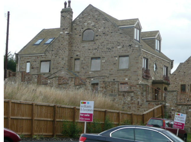
HOUSES AT HILL TOP MOOR TO NORTHERN BOUNDARY
