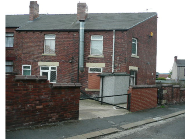
ENTRANCE TO HAVELOCK STREET EAST
