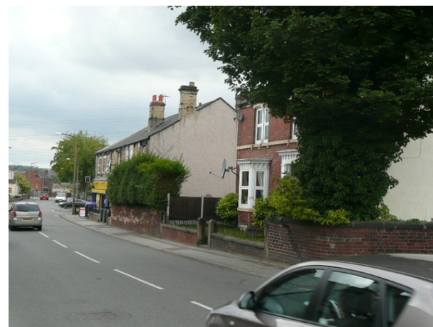
EXISTING HOUSES LOOKING WEST DOWN SNAPE HILL
