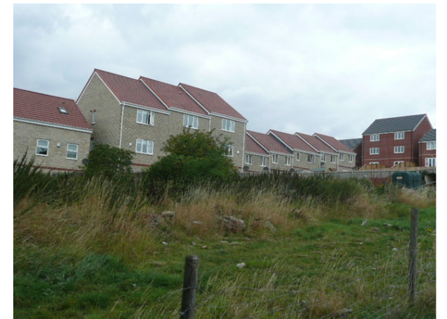
HOUSES OFF VERONA RISE ADJACENT WESTERN SITE BOUNDARY.
