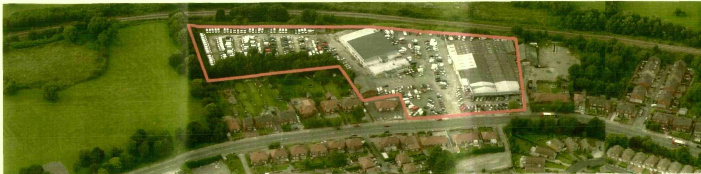
Aerial View of Site
